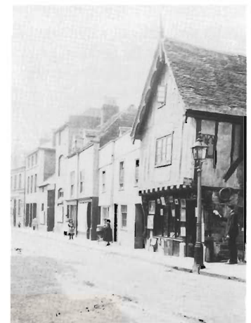
Bourne Street, Hastings Old Town.
