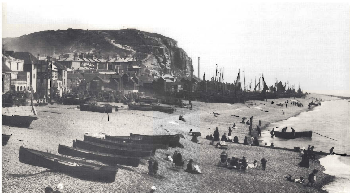
The fishermen's Stade at Hastings. The wholesale fishmarket is centre left, with the netshops stretching along under the East Cliff, and the fishing fleet on the brow of the beach.
